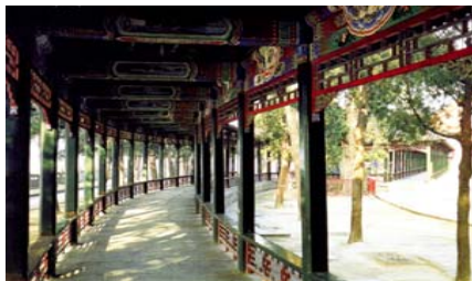
Long Corridor - traditional architecture
