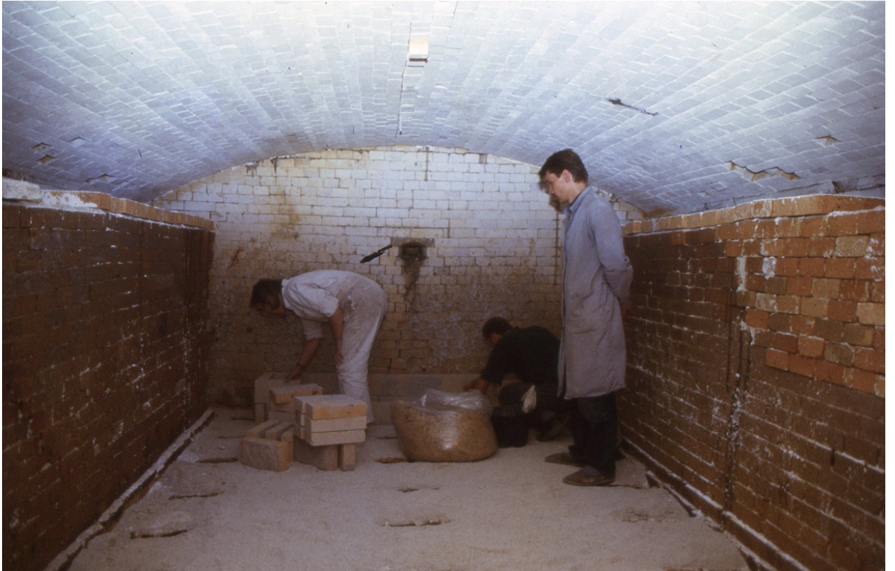
Panevėžys Glass Factory. Inside of the kiln. 1992
