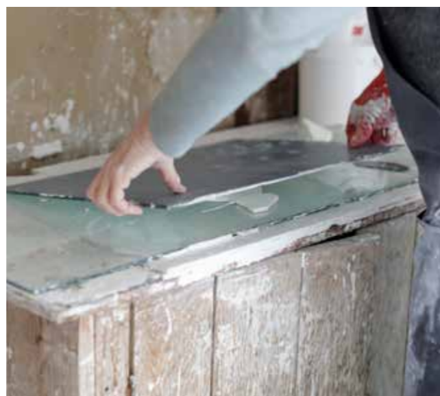
4 A second sheet of glass is placed on top until the plaster is set. I rest the glass on three spacers, each measuring approx. 1cm thick. The size of the spacers determines the thickness of the plaster.
