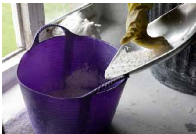
15 The plaster is added gradually to the measured water.
