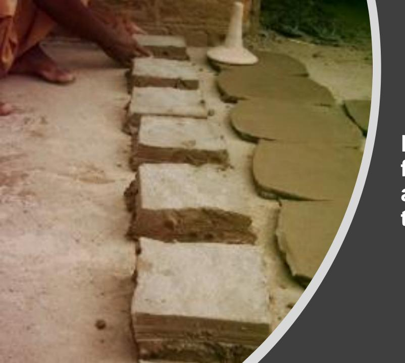
Placed on mud floor in a line and applying sand to the top surface.
