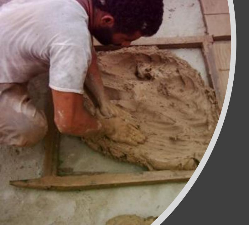
Clay is pressed by hand into large sized slabs.
