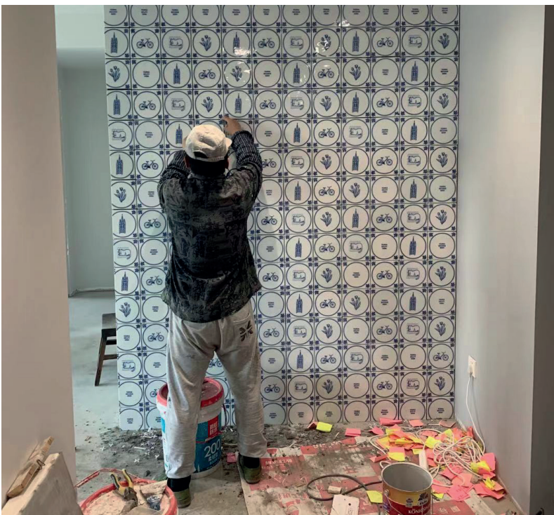
Applying the Delft blue tiles to Terra's entrance
