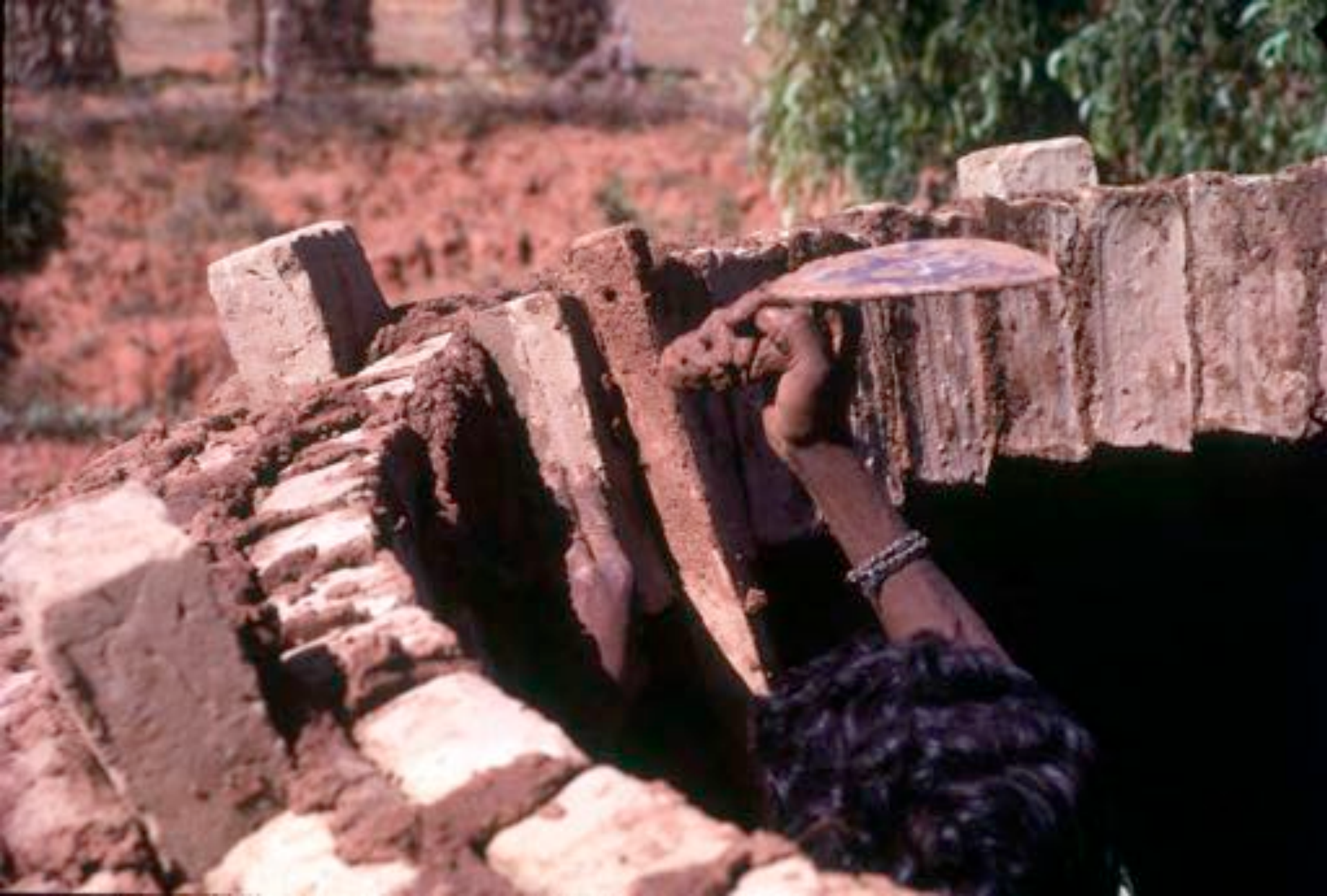
Note the saw-toothed edge of the upper dome layers. Each brick hangs on the previous course as well as on the adjacent brick from the same course.
