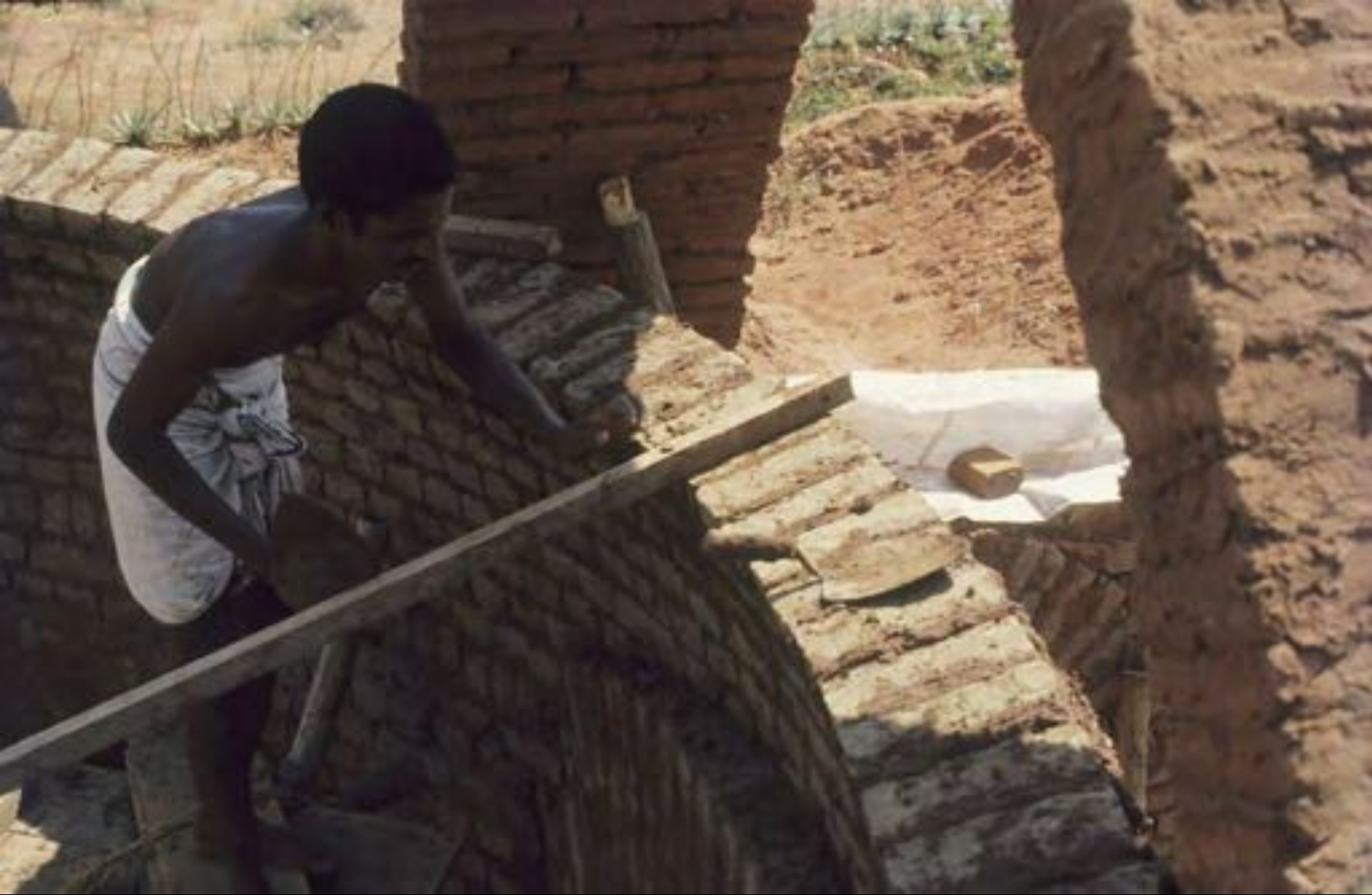
Beginning the 5 m dome. This is the first dome that this mason has ever built.
