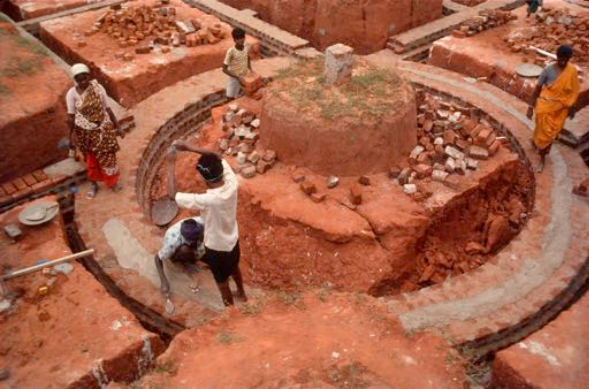
Foundations are in fired brick and lime mortar.
