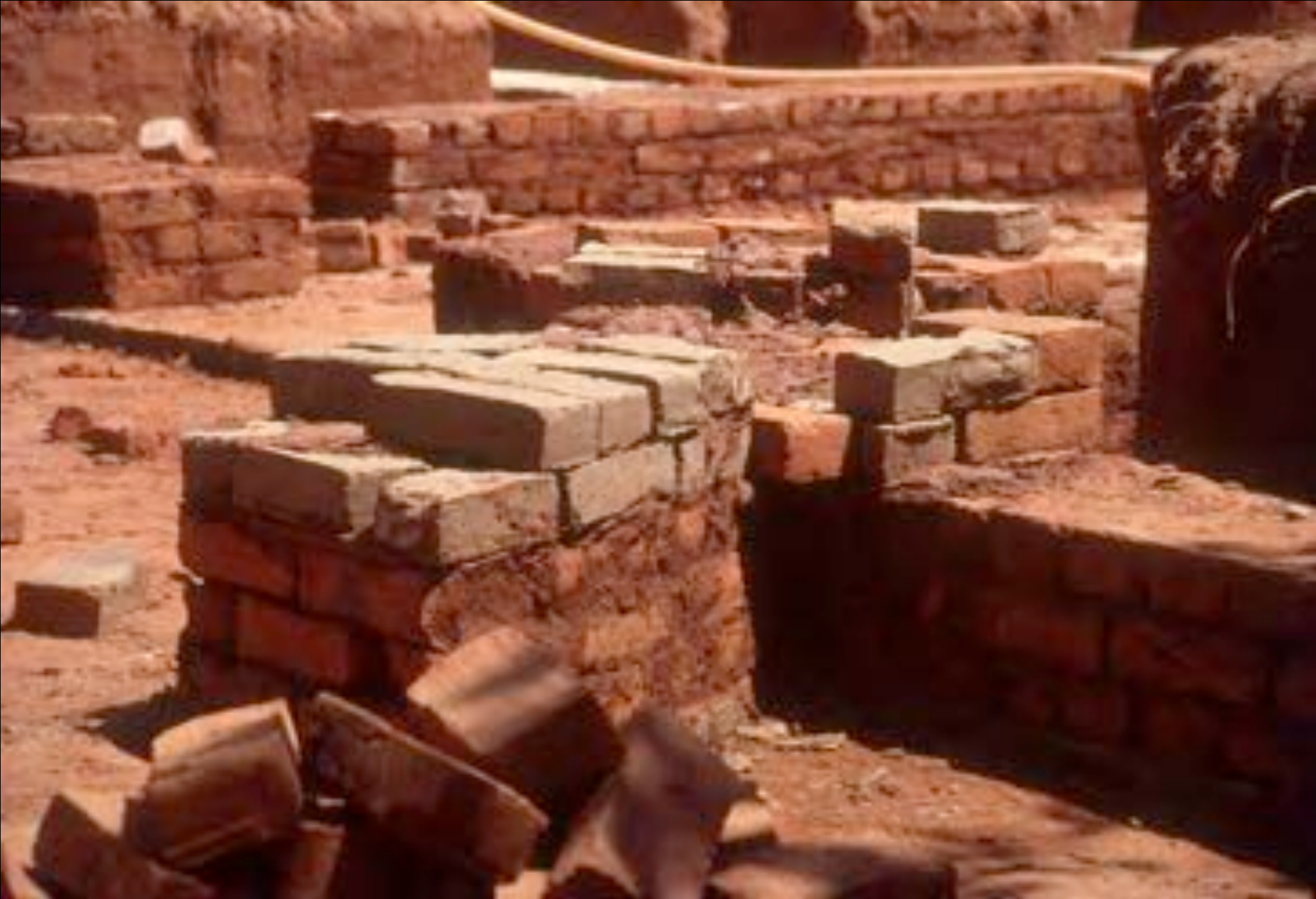
Mud brick begins three brick courses above the floor level. Experience had shown that the lower wall tended to be under-fired.
