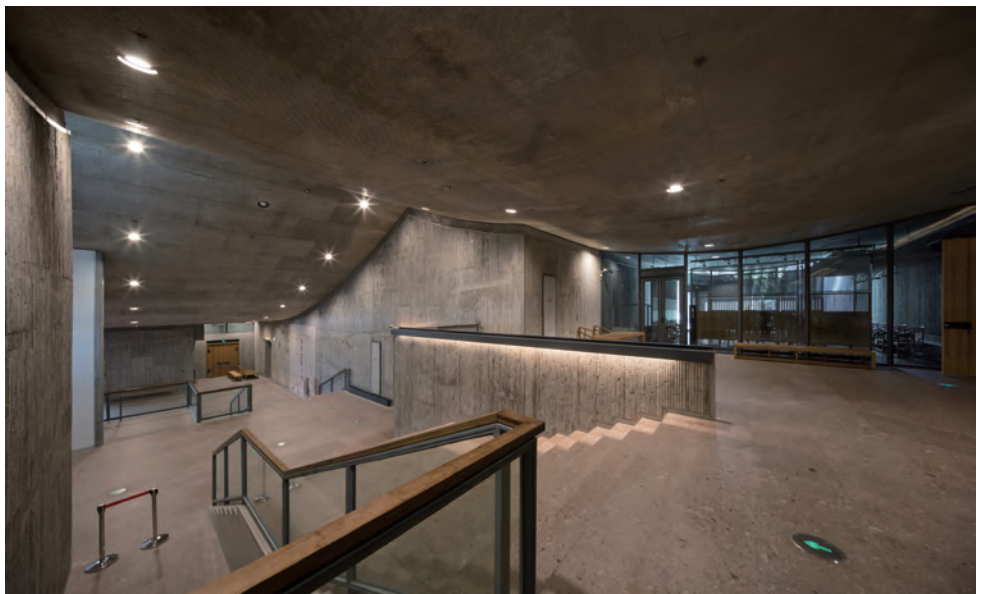
Bamboo formwork gives texture to concrete at Fuchun Cultural Complex © Lv Hengzhong
